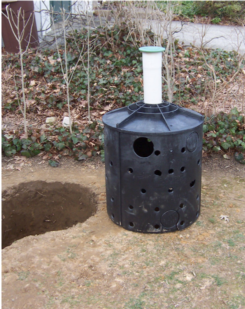
ROCK INFILTRATION CHAMBER - DOWNSPOUT CONNECTION
