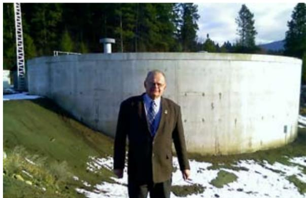
“This covered water storage facility is another step in providing safe, clean water to the residents of Creston,” Mayor Joe Snopek said after a recent inspection of the new Crawford Hill Reservoir. A total of 800 cubic metres of concrete was used to build the reservoir, which can hold up to 4.5 million litres of water.
