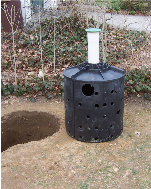
ROCK INFILTRATION CHAMBER - DOWNSPOUT CONNECTION
