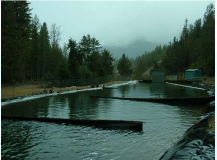
Arrow Creek Raw Water Supply
