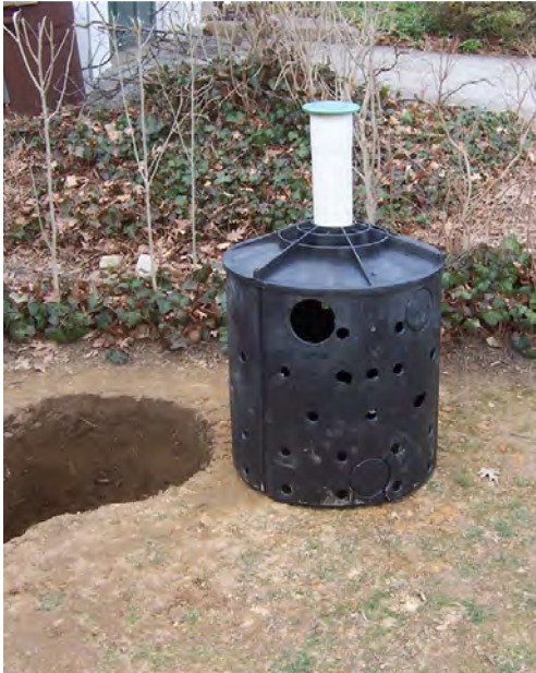
ROCK INFILTRATION CHAMBER - DOWNSPOUT CONNECTION
