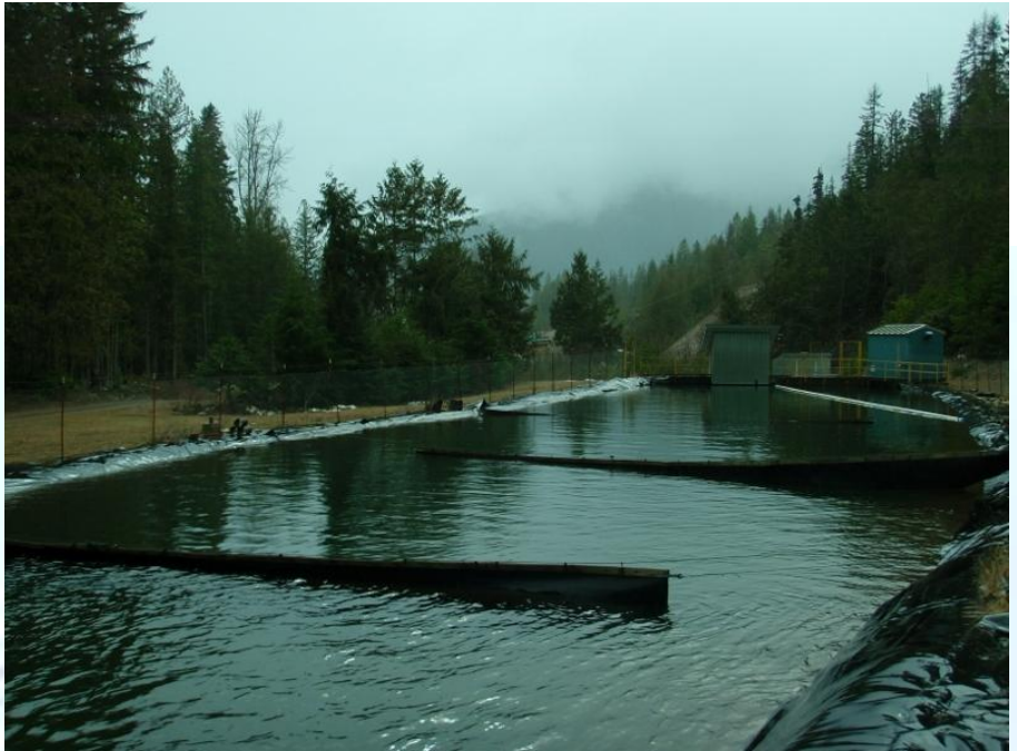
Arrow Creek Raw Water Supply
