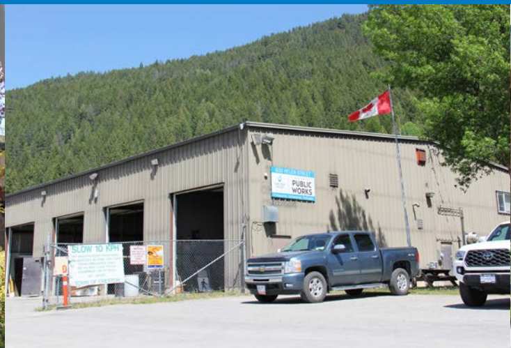
Public Works Building
