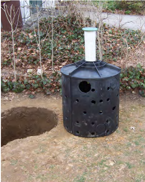
ROCK INFILTRATION CHAMBER - DOWNSPOUT CONNECTION
