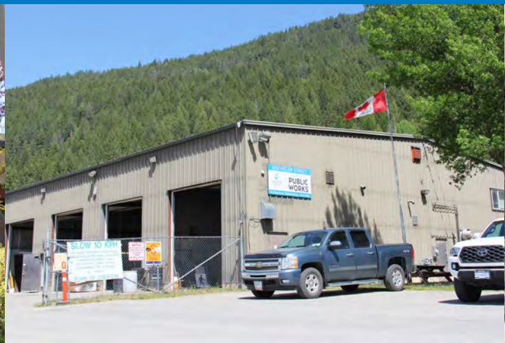
Public Works Building
