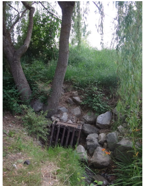
Figure 4: 5th Avenue Culvert
